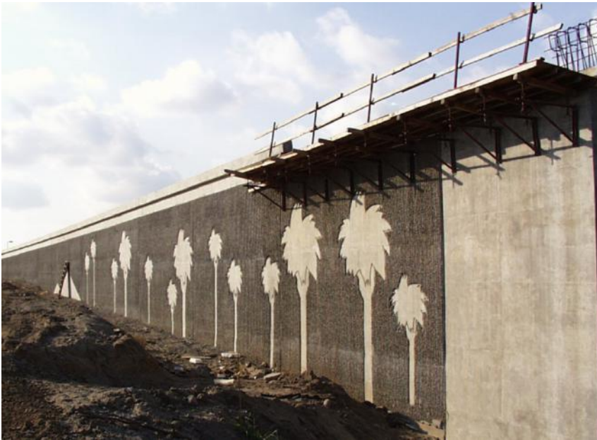
Figure 3.19: Photo. Cast-in-place facing. Photograph courtesy of DYWIDAG-Systems International.
