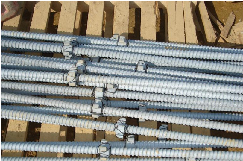
Figure 3.7: Photo. Typical steel centralizers attached to HBSNs. Photograph courtesy of Schnabel Engineering.
