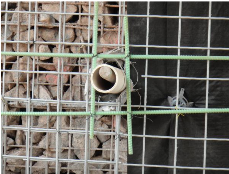
Figure 3.18: Photo. Shotcrete reinforcement including WWM and waler bars. Photograph courtesy of Ryan R. Berg & Associates, Inc.
