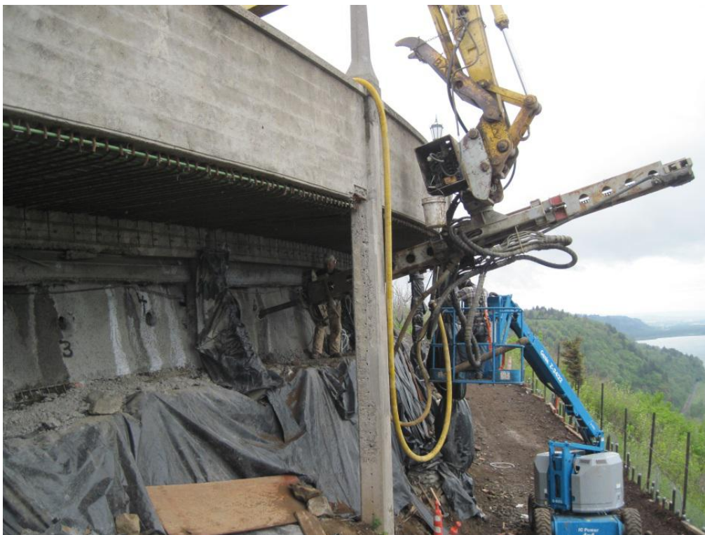
Figure 3.15: Photo. Drilling nail holes. Photograph courtesy of Barry Siel, FHWA.
