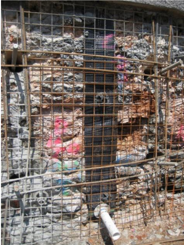
Figure 3.12: Photo. Strip drain prior to initial shotcrete placement. Photograph courtesy of Schnabel Engineering.
