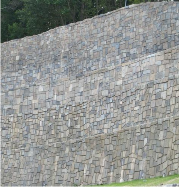
Figure 3.21: Photo. Sculpted wall facing. Photography courtesy of The Collin Group, Ltd.
