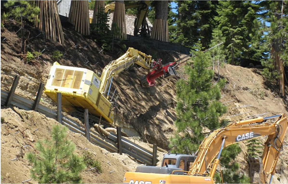
Photo 3. Soil nail launcher operating on slope by Lake Tahoe in El Dorado County, CA (photo courtesy of Colby Barrett, Soil Nail Launcher, Inc.).
