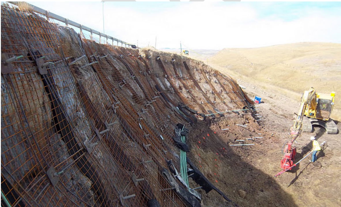
Photo 4. Soil nail slope in Wyoming with nail face plates and wire mesh in preparation for shotcrete application (photo courtesy of Colby Barrett, Soil Nail Launcher, Inc.).
