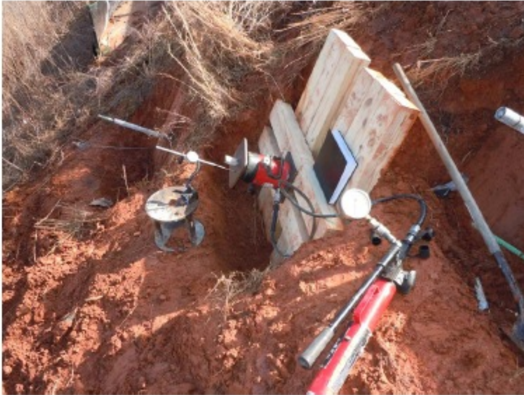
Figure 3: Middle Row Test Nail
