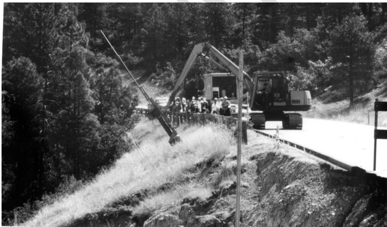
Photo 2. Excavator-mounted soil nail launcher reaching over guard rail to repair a failing slope (USFS, 1994).
