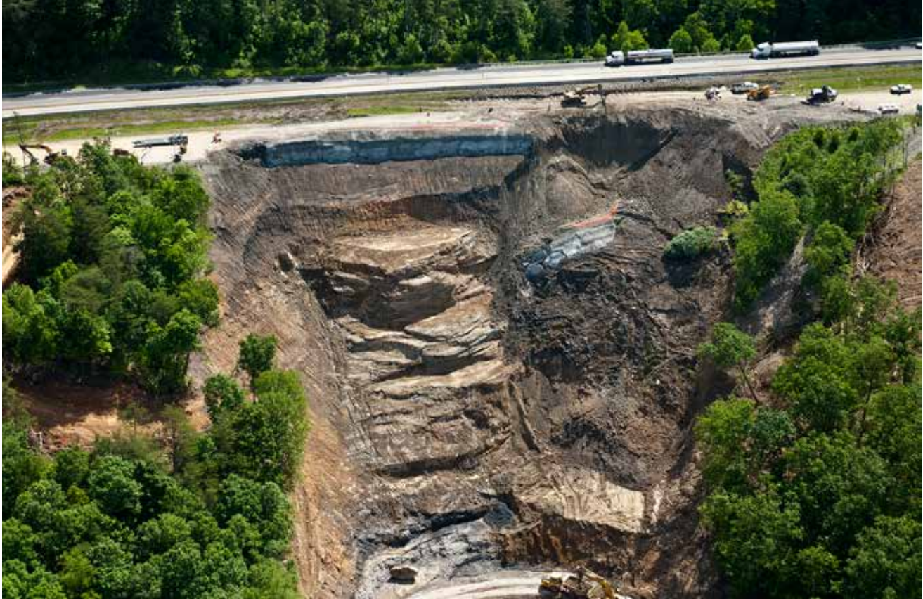
Launched soil nails used to prevent the regression of a large landslide in northern Tennessee (2012). Note the launcher at the top of the photo for scale. (Photo courtesy Tennessee DOT.)
