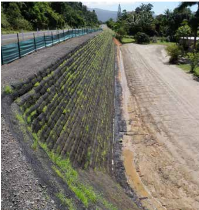
Completed launched soil nail geosynthetically confined soil wall in Cairns, Australia (l) immediately after wall construction, and (r) vegetated-face 18 months later. (Photo courtesy Hiway Geotechnical Ltd.)
