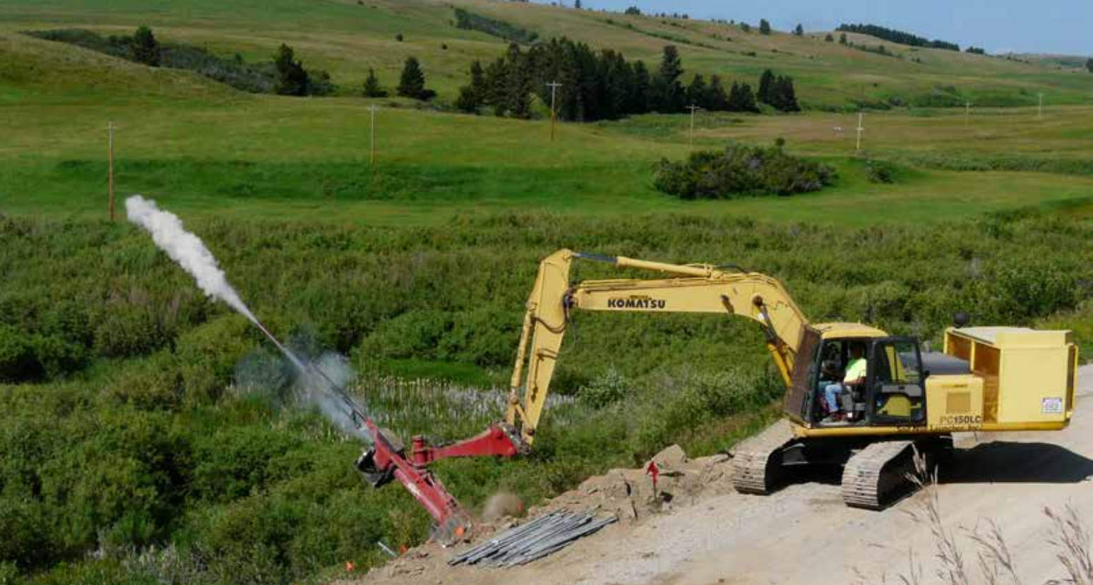
Riparian landslide repair using pressure-grouted launched soil nails for Western Federal Lands Highway Department.
