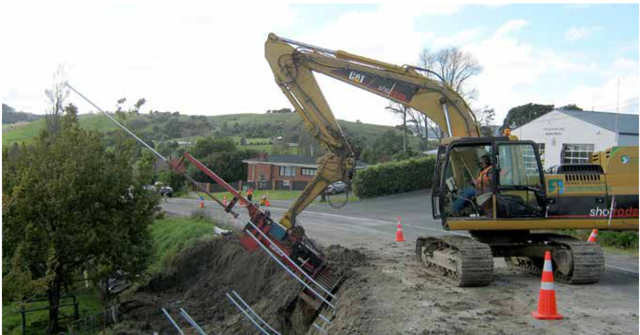
Launched soil nail shoring to support a roadway in Northland, New Zealand. (Photo courtesy Hiway Geotechnical Ltd.)
