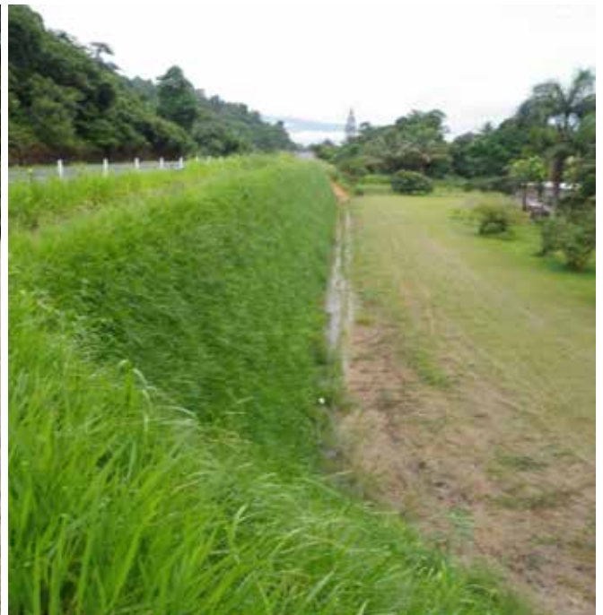
Completed launched soil nail geosynthetically confined soil wall in Cairns, Australia (l) immediately after wall construction, and (r) vegetated-face 18 months later. (Photo courtesy Hiway Geotechnical Ltd.)
